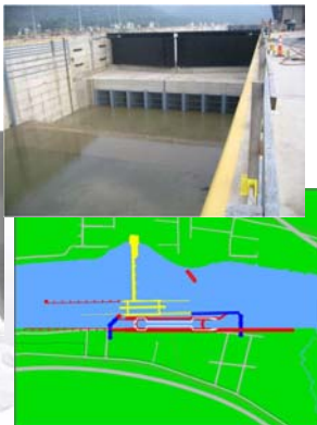
Through-the-Sill Design Reduced Cofferdam Size
