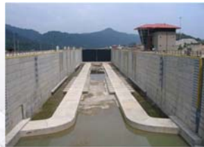
In-Chamber Longitudinal Culvert System
