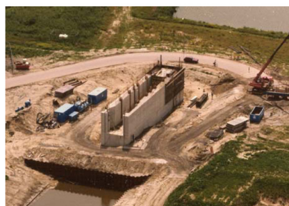
Fig 4.3 : Whole lock structure to be immersed - Almere Haven (NL)
