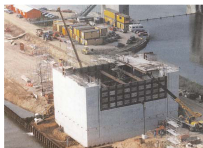
Fig 4.4 : Upper lock head structure to be immersed - Lith (NL)
