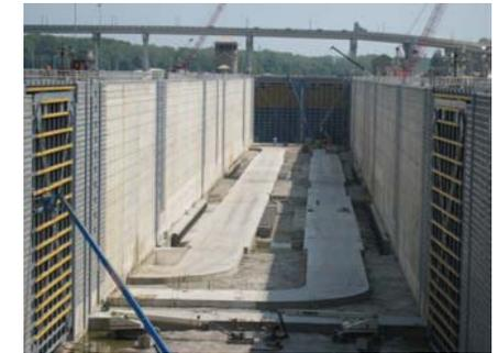
Fig 2: In-chamber longitudinal culverts, McAlpine Lock
