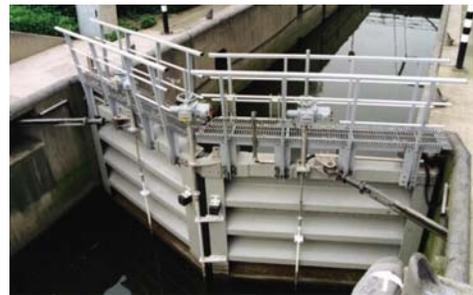
**Fig. 1.** FRP gate of a lock near Werkendam
