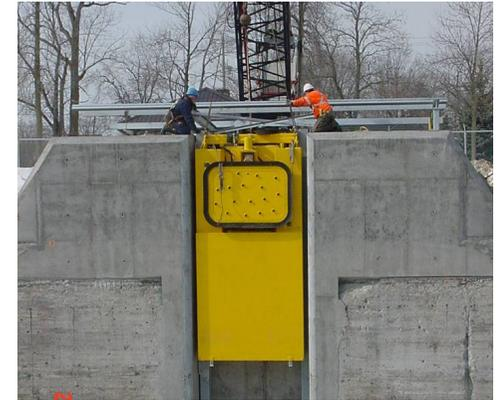
Figure 1 - HFM Flotation Unit
