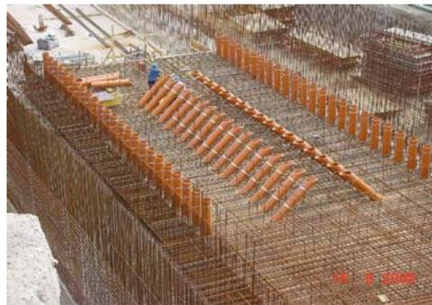
Picture 1: Permanent formwork for the pressure chamber of Sulfeld lock
