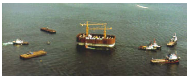
Fig. 7.15: Alignment with Winch Lines and Tugs
