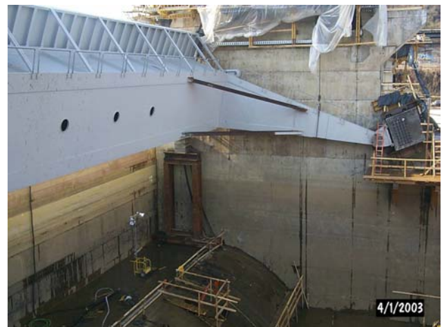
Fig. 7.23: Braddock Tainter Gate – Final Adjustment “In-the-Dry”
