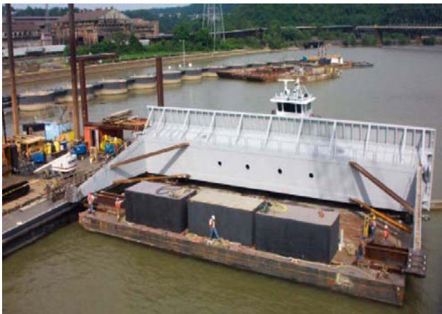
Fig. 7.20: Tainter Gate Transported by Barge to Braddock
