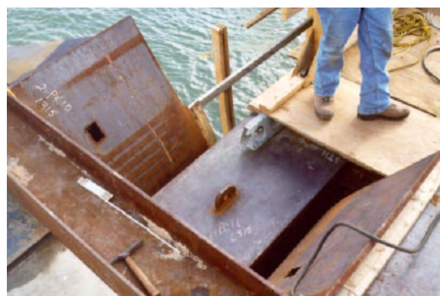
Fig. 7.18: Horned Guide w/ Mated Section
