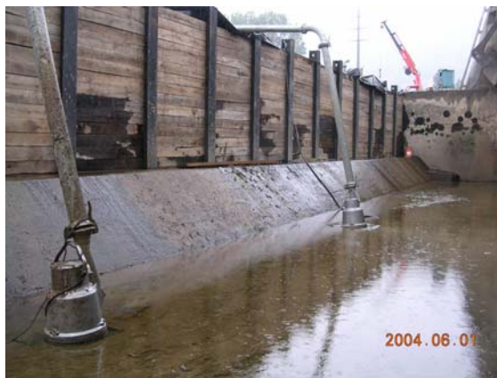
Fig. 5.21: Beam Bulkhead System
