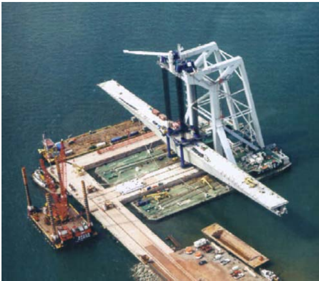
Fig. 7.7: Catamaran Crane Barge of 8500 tons capacity, ERDC/GSL TR-00-2
