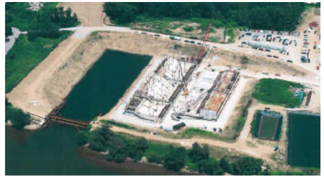
Fig. 7.10: Braddock 2 Level Graving Dock at Leetsdale
