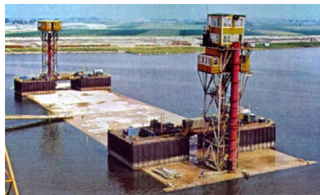
Fig. 7.16: Immersed Tube Bridge Segment w/ Spotting Towers (EM1110-2-2611, page C-9)
