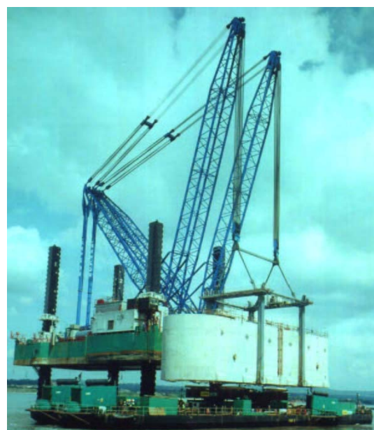
Fig. 7.6: Jackup Barge with a Heavy Lift, ERDC TR-02-22
