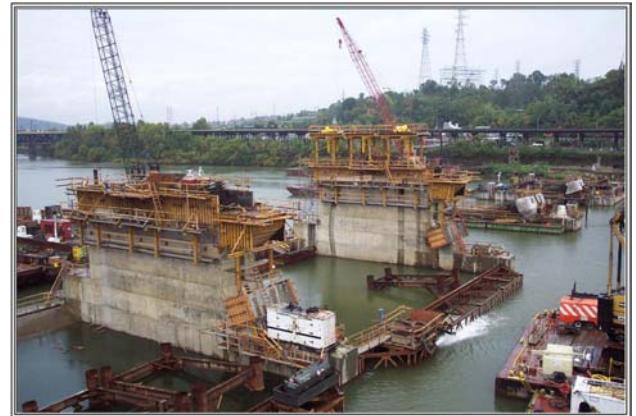
Fig. 7.22: Tainter Gate Bulkheads in Place to Dewater the Gate Bay
