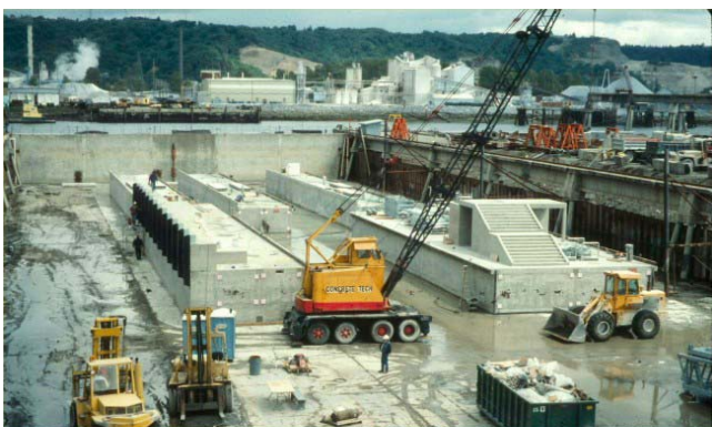
Fig. 7.8: Concrete Tech Graving Dock w/ Port of Bremerton Floating Dock
