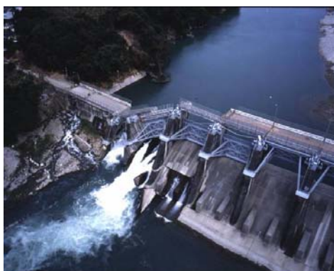
Fig. 5.9(a): Collapse of the Shih-Kang weir (Taiwan)
