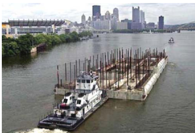
Fig. 7.3: Braddock Dam Float-in Tainter Gate Foundation
