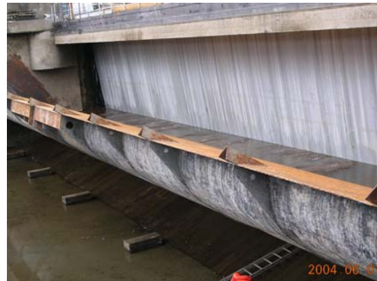
Fig. 5.18: Bulkhead needles supported by an upper beam
