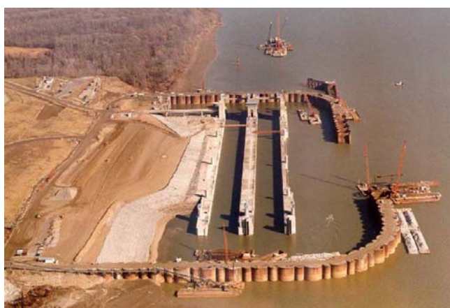
Fig. 7.2: Olmsted Locks Cofferdam being removed
