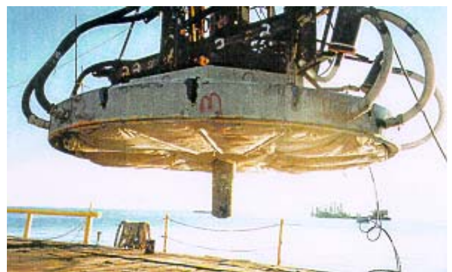
Fig. 7.12: Grout Bag with Grout and Vent Tubes Attached
