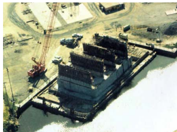
Fig. 7.4: Montezuma Slough Salinity Barrier Precast Construction on a Barge
